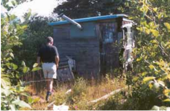
Figure 27: A small one room cabin has been constructed on the abandoned rail line. It overlooks the pond on the Melanson Property, and has a bed and stove. There is no sign of current use, although materials used in construction are quite modern.
